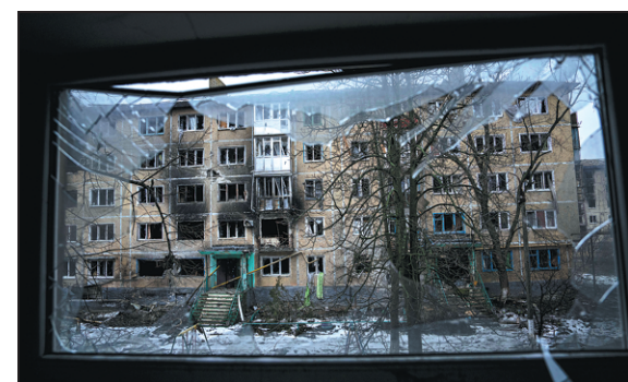
A badly damaged residential building is seen through a broken window in Vuhledar, Donetsk, on Saturday. EVGENIY MALOLETKA / AP
